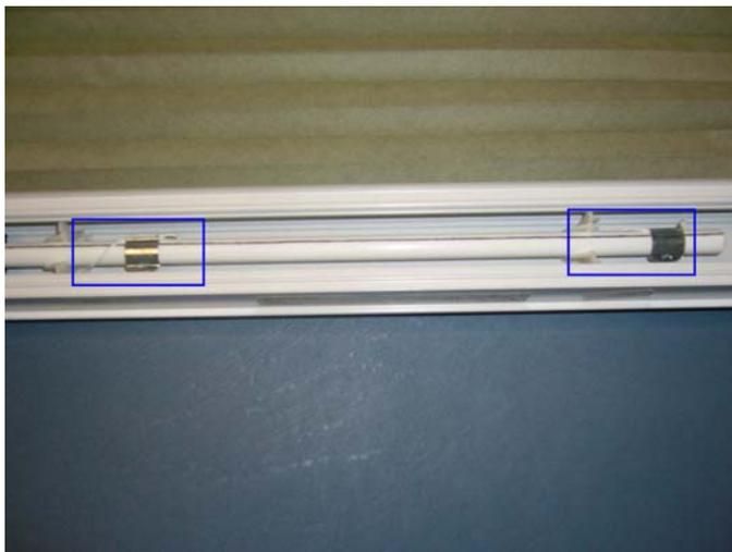
5. If the C-clips are not positioned evenly in the headrail, slide the clip away from the cradle to raise the shade or toward the cradle to lower the shade.
