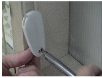
2. Remove shade from installation brackets using a flathead screwdriver. Insert tip of screwdriver between the back of the headrail and the bracket.
