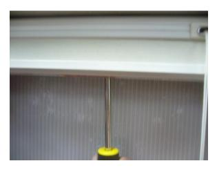
3. Unscrew the top joiner ball. Set aside danskord (thick rope cord). Untie joiner ball knot. Remove joiner ball and washer.
