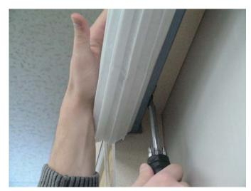
**6.** Check the brackets to ensure that they are a minimum of 3" in from each end. If not, reposition the brackets.
