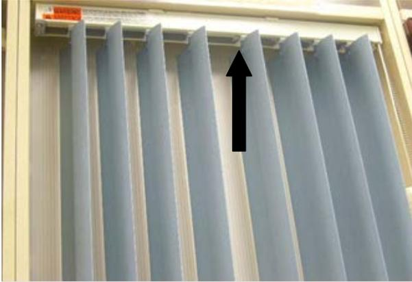
2. Rotate the louvers open and slide a hard plastic card between the louver and the long side of louver stem. Push card and louver up toward top of louver stem. This will unseat the louver from the louver stem.
