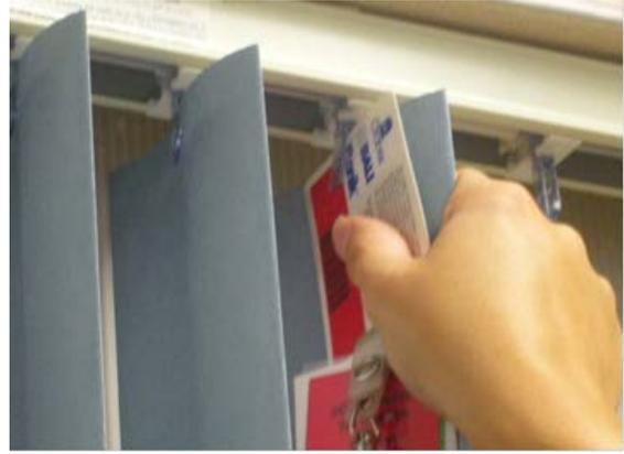
3. Remove the louver by pulling down on both louver and plastic card at the same time. Lay the louver on a clean flat surface. Repeat for all louvers.
