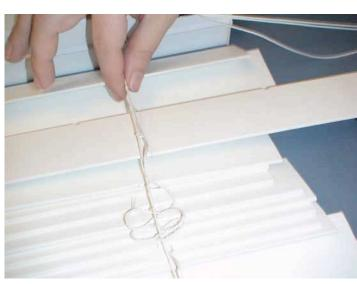
**7.** Raise and lower the blind with the slats in the open position to make sure it operates properly.
